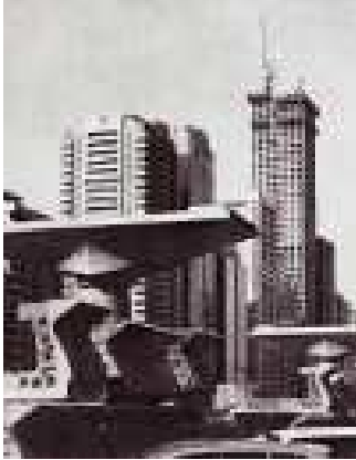
6. Martin BECKA Subway Construction
