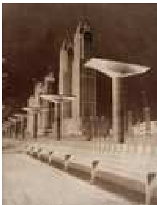
8a. Martin BECKA Dubai Media City Area, Al Kazim Towers nég.
